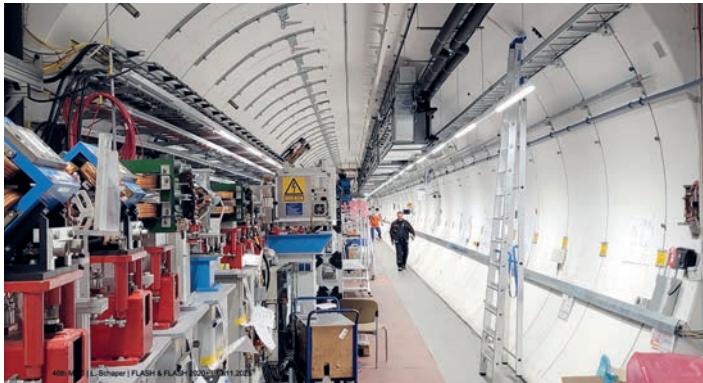
Figure 1 A glimpse into FLASH1 as seen from the beam dump looking upstream towards the photoinjector. Left: View of the tunnel after removal of the old beamline and after infrastructure refurbishment. Right: Newly installed FLASH1 beamline.
