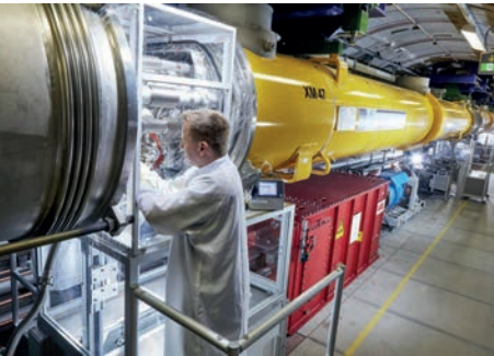
The Long Installation and Maintenance Period enabled major work on the European XFEL linear accelerator.
