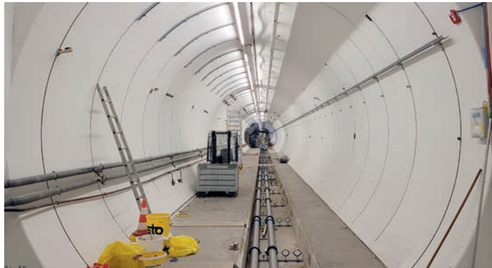
Figure 1 A glimpse into FLASH1 as seen from the beam dump looking upstream towards the photoinjector. Left: View of the tunnel after removal of the old beamline and after infrastructure refurbishment. Right: Newly installed FLASH1 beamline.
