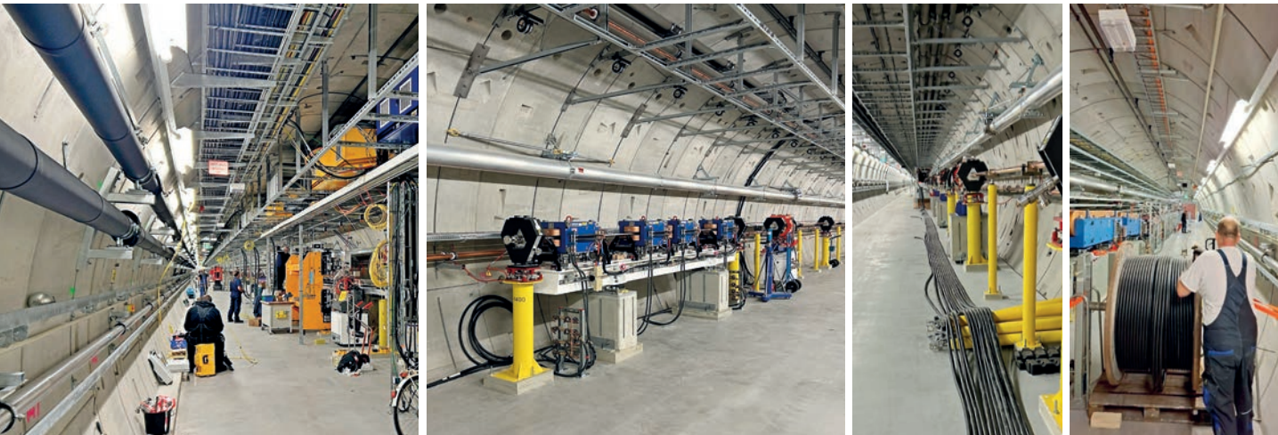
Figure 2 Left: Installations behind the SASE2 section in the XTD1 undulator tunnel. Centre: New chicane in the XTD2 undulator tunnel. Right (two pictures): Cabling work in the XTD4 undulator tunnel.
