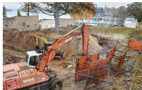
Start of the CTA SDMC construction work
