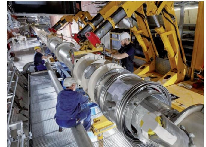
In late 2020, the last of the superconducting ALPS magnets were installed in the tunnel. Meanwhile, the entire chain has been cooled to  $-269^{\circ}\text{C}$  with liquid helium.
