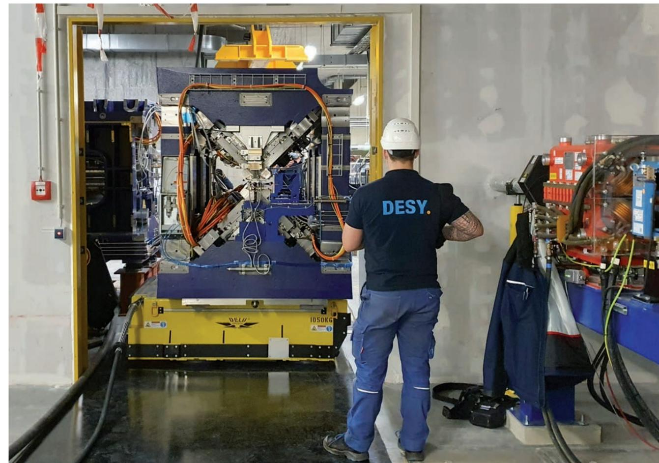
Figure 2 Transport of one of the APPLE-X undulators in the European XFEL undulator tunnel
