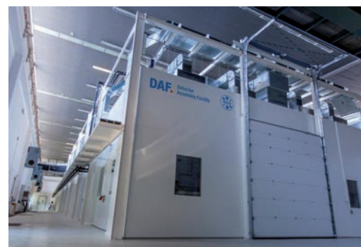
DESY’s Detector Assembly Facility is complete.
