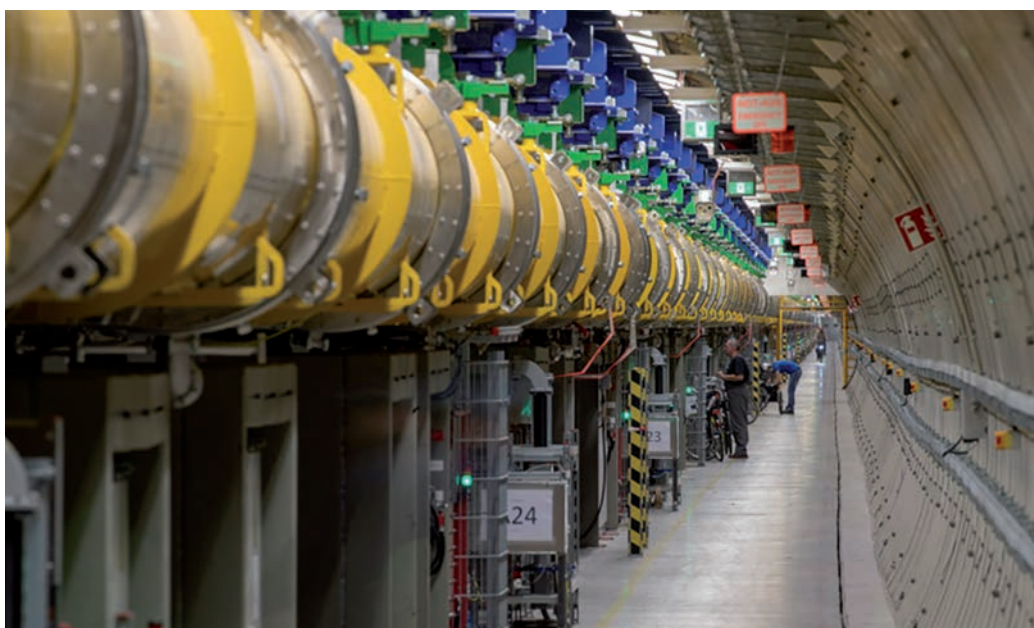
Figure 1 Maintenance work in the European XFEL accelerator tunnel
