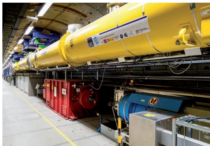
View into the tunnel of the 1.7 km long superconducting linear accelerator of the European XFEL
