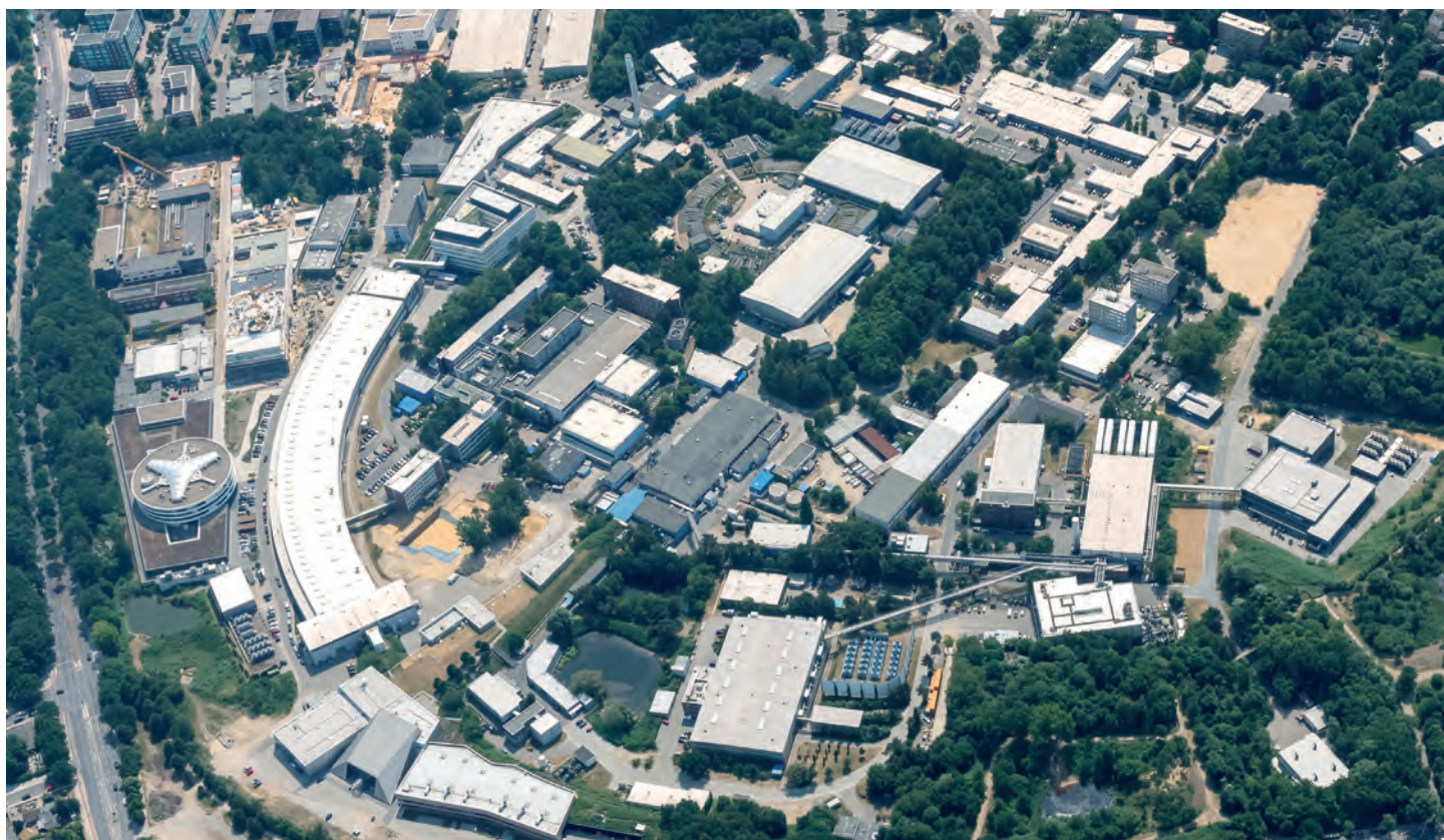
The DESY site in Hamburg with the new CSSB building and the construction sites for the Max Planck Institute for the Structure and Dynamics of Matter (MPSD) and the Centre for X-ray and Nano Science (CXNS) on the left and right side of the curved PETRA III experimental hall 'Max von Laue' in May 2018.
