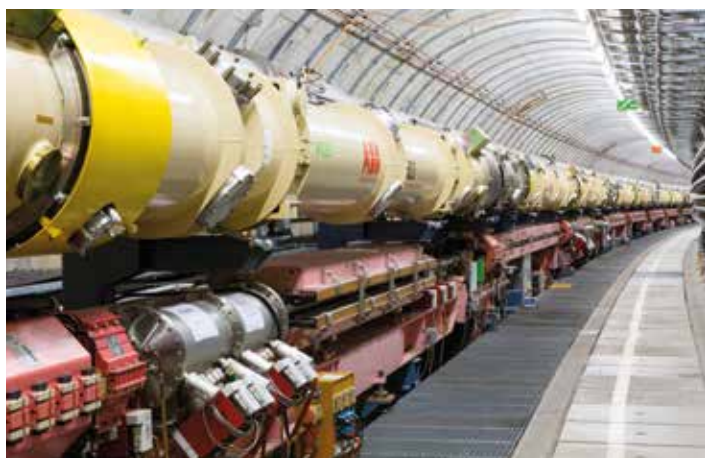
The HERA accelerator tunnel
