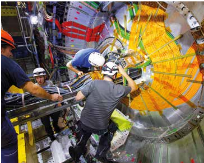
Figure 1 Installation of the vertex detector into the Belle II experiment at the SuperKEKB collider in Japan in November 2018
