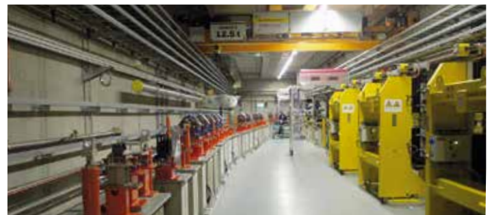
Construction of the beamline (left) connecting the FLASHForward experiment to the FLASH accelerator
