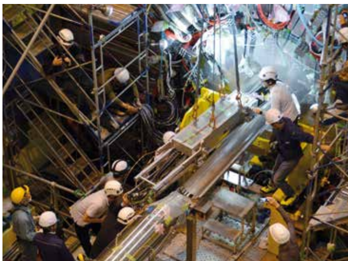
Figure 1 Installation of the BEAST II detector in the Belle II experiment at the SuperKEKB collider at KEK in Japan (November 2017)
