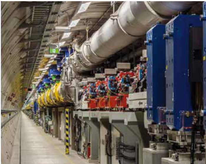
View into the European XFEL accelerator tunnel
