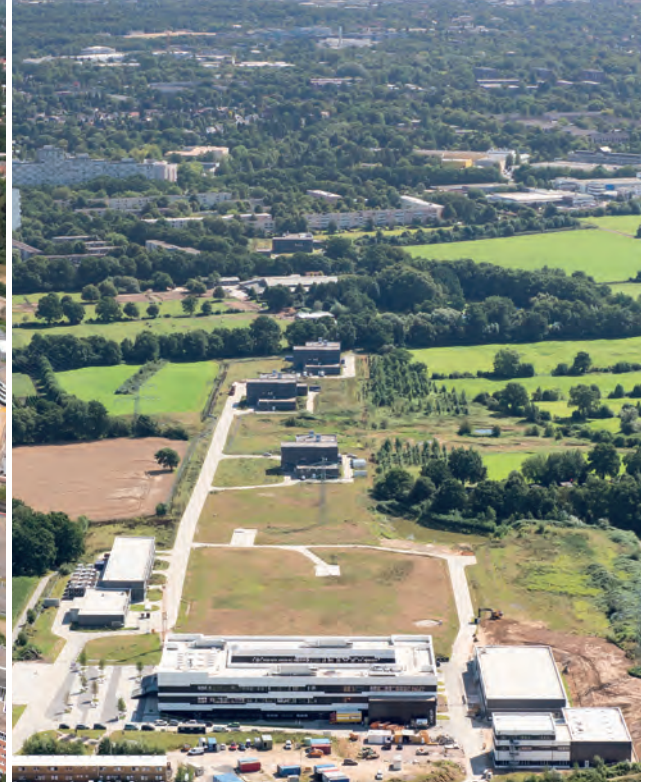
The European XFEL site (Schenefeld) with the DESY site in the far background. The 3.4-kilometre-long European XFEL runs from DESY to the underground experimental hall in the main building (foreground).
