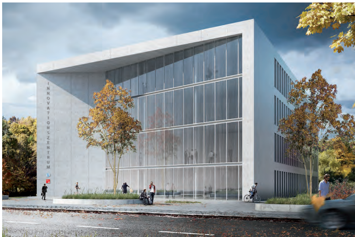
Figure 1 Architect concept of the Innovation Centre to be constructed at the Luruper Hauptstraße on the campus and adjacent to the CFEL building and PETRA III experimental hall 'Max von Laue' (DFZ Architekten GmbH).
