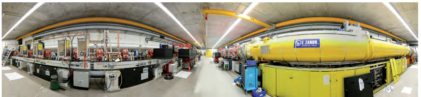
Figure 1 Overview of the European XFEL injector. Left: warm beamline. Right: electron gun and accelerator modules.
