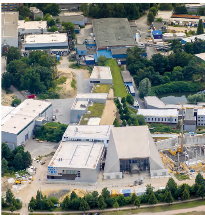
The FLASH facility with the two experimental halls in the foreground
