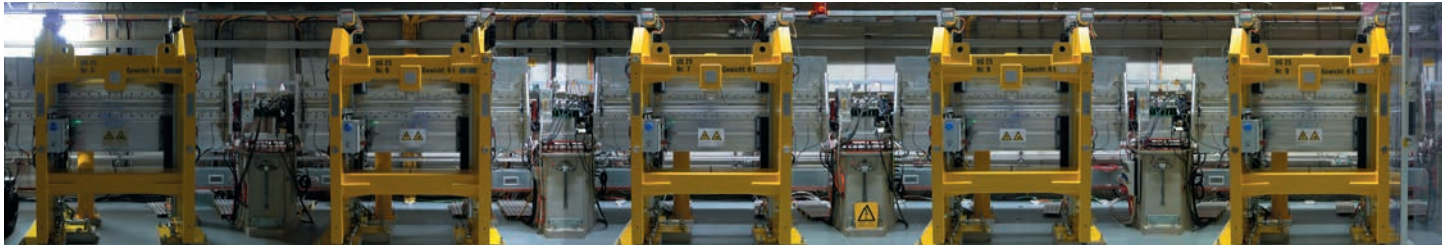
Figure 1 Part of the FLASH2 SASE section comprising 12 undulators and corresponding intersections
