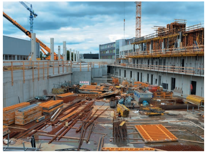
Figure 8 Civil engineering of hall east (August 2014).
