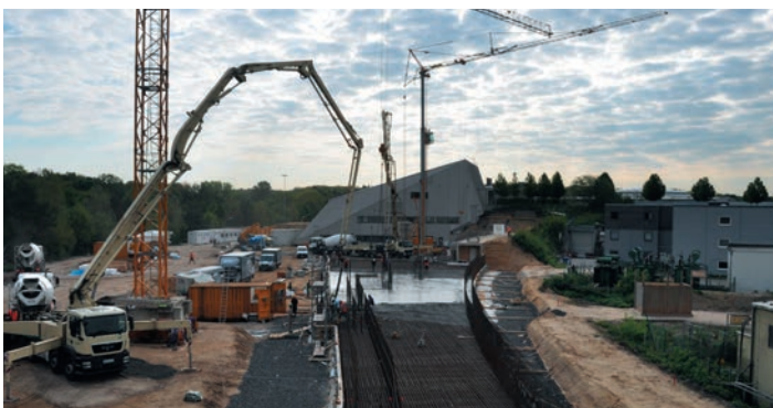
Figure 7 Casting of the base plate for hall north (April 2014).
