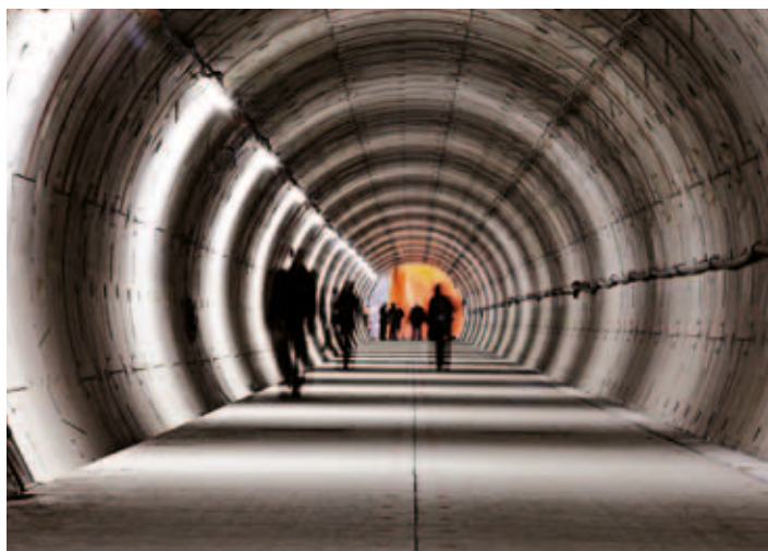
The accelerator tunnel for the European XFEL
