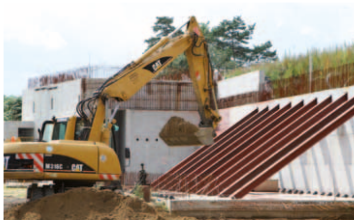
Construction site of the FLASH II main tunnel
