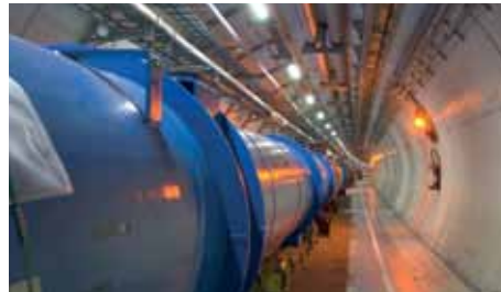
View into the LHC tunnel (Photo: CERN)
