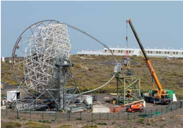
Figure 2 Replacement of the MAGIC-I camera
