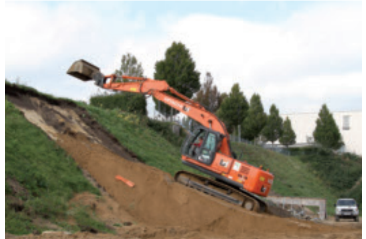
First digging at the FLASH accelerator tunnel
